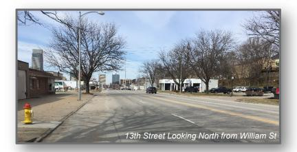
Sidewalk zone width is approximately 20' on each side and is distributed among the furnishing, pedestrian, and frontage zones like the section to the south. There are multiple locations of broken or uneven sidewalks on the east side of the street as well as one area of brick sidewalks on the west side north of Pacific Street.
